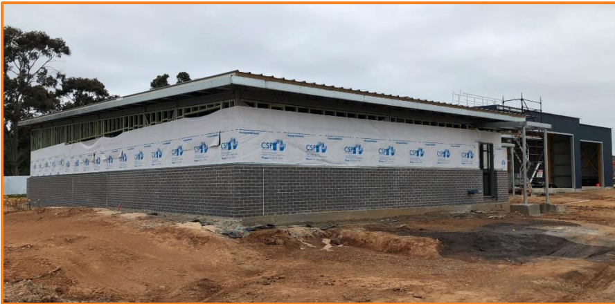
VICSES Wangaratta construction underway at 36 Handley Street, Wangaratta – October 2020.
