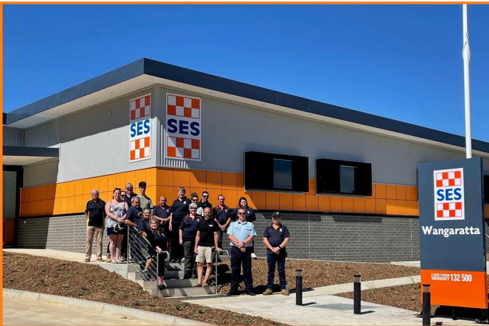
VICSES Wangaratta construction completed at 36 Handley Street, Wangaratta – December 2020.
