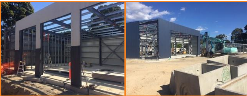
Construction underway for the new Knox Unit – progress as at February 2021
