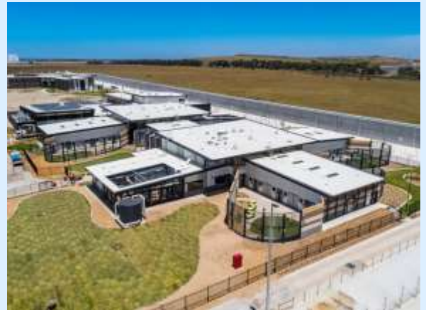
DPFC 106 beds and supporting infrastructure aerial view
