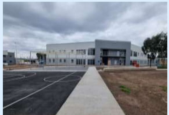
Marngoneet Correctional Centre – accommodation unit
