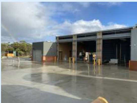
St Leonard's Fire Station
