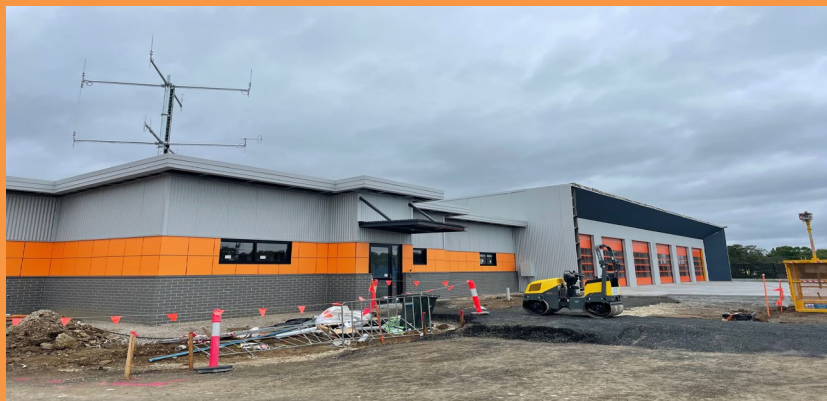
VICSES Cranbourne – External Pavement works progressing
