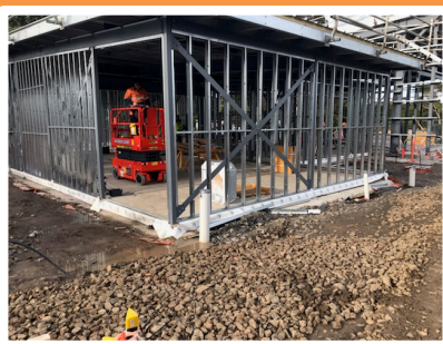
Structural Steel, roof and internal framing
