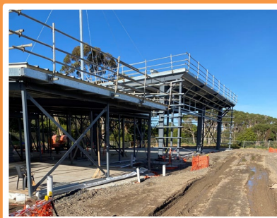
Structural Steel, roof and internal framing
