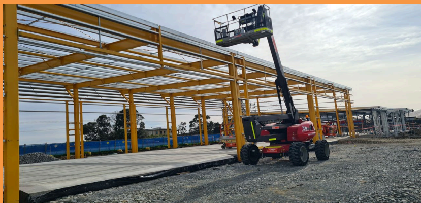
SES Cranbourne – Steel Structure erection completed
