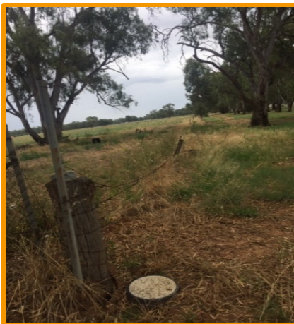
Service connections installed
