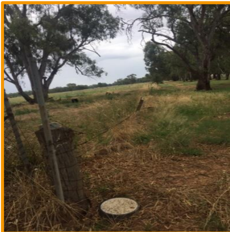
Service connections installed
