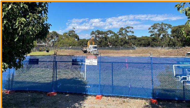
VICSES Fawkner (Broadmeadows) Unit construction commencement
