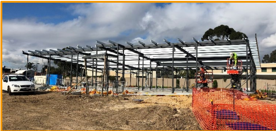
VICSES Fawkner (Broadmeadows) Unit construction
