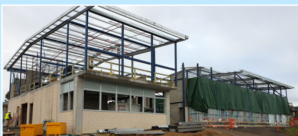
New accommodation at Middleton prison in construction with the modular cells under tarpaulins until the building is watertight.
